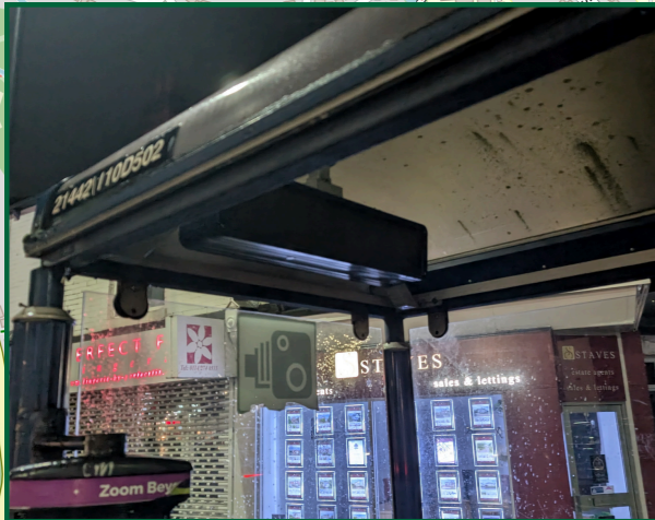
Secured repairs to damaged bus stops throughout our area, including in Woodseats, Meadowhead and Norton Lees
